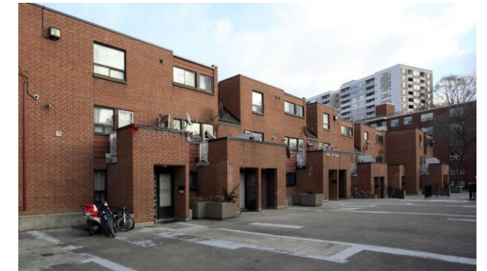
Fig. 5. Existing construction materials can be reused for the proposed redevelopment.
